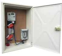
Typical layout within the outside box. Note: Cable entry and exits at the bottom of the box. Customer cable may also enter through a predrilled hole at the bottom right-hand of the hox.
