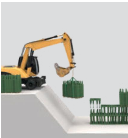
Assembly inside the excavation pit
