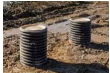
Temporary construction site cover for extension pipes
