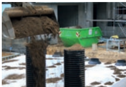
Purpose of temporary construction site covers when backfilling
