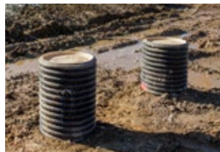
Temporary construction site cover for extension pipes
