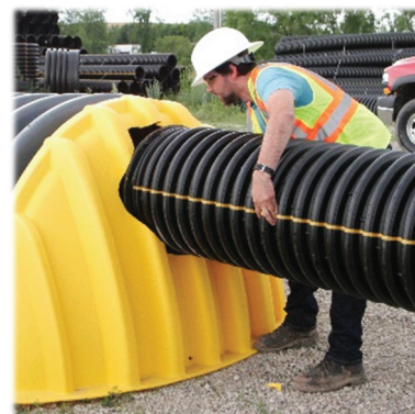
Figure 4: Inserting the Pipe
