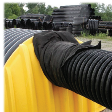
Figure 6: Proper Geotextile Placement
