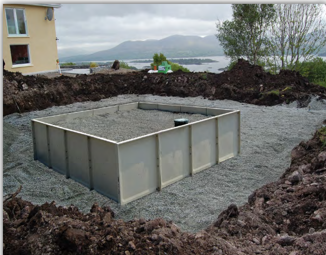
Sandcel during installation
