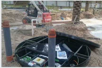
▶ Treatment plant during installation.
