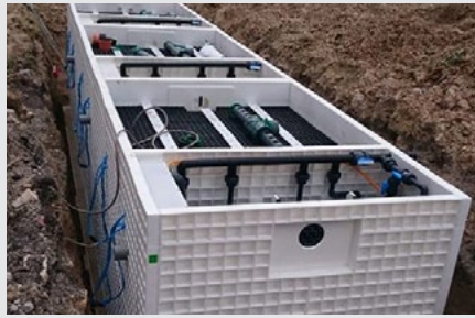
▶ Treatment plant during installation.
