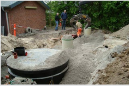
▶ Installation with combined GRP settlement and buffer tanks.
