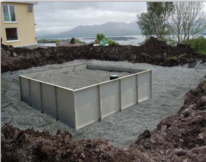
Sandcel during installation
