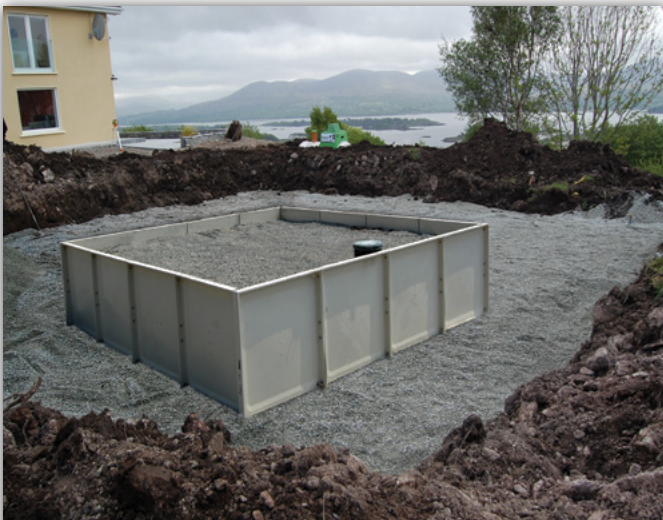
Sandcel during installation
