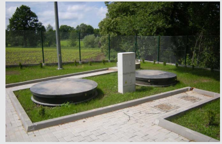
▶ Remote settlement and buffer tanks to suit a site with restricted space.
